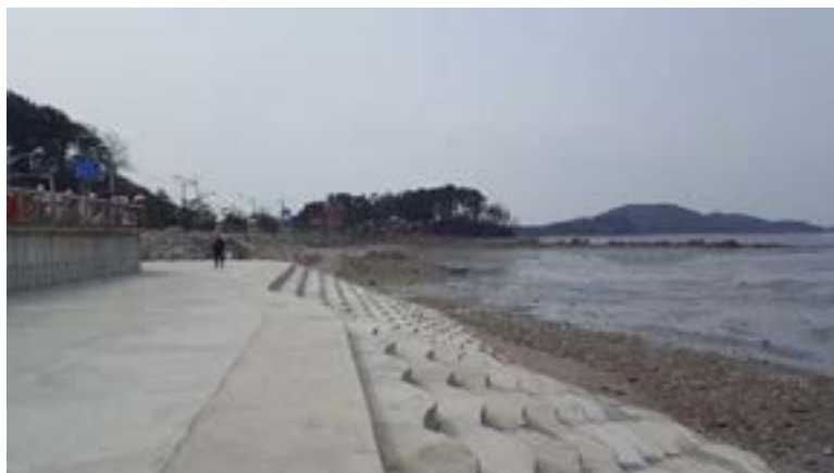
Figure 6. Recently constructed small embankment on the beach
