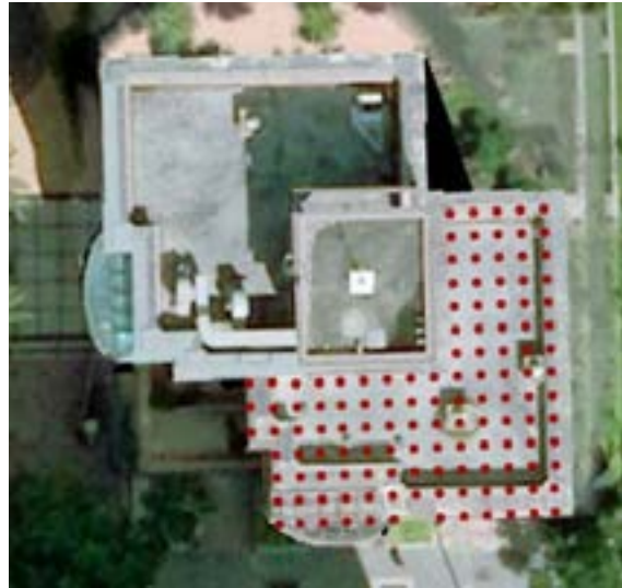
(b) the majority-based results are affected by other objects (e.g., water tower) and broad parapet walls
