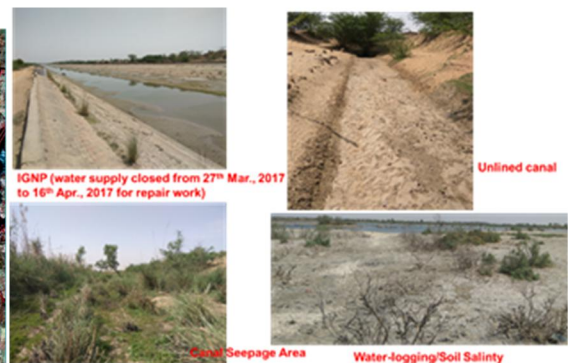
Figure 4: Field photographs showing sub-surface seepage and water-logging/ Salinity.
