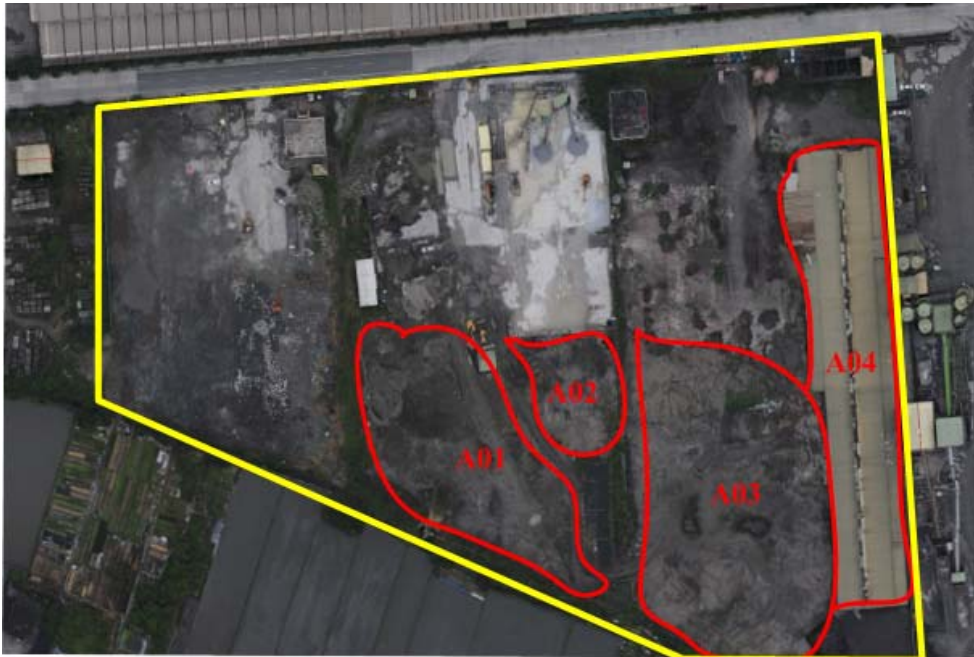
Figure 10 UAV photo of the illegal dumping site (Tsai and Chen, 2014)
