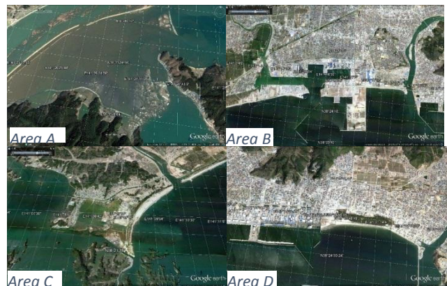
Figure 6: Damage area due to the disaster on 11 th March 2010
