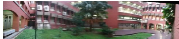
Figure 14 first floor of classrooms
