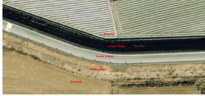
(a) High resolution orthoimage showing the multiple levee components.
