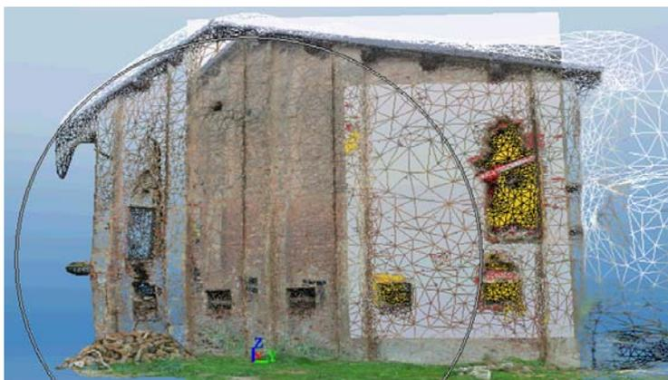
Figure 5: Wire-mesh model of the building shown in Figure 3C, with the colored point cloud, as well as detected damage (windows/holes) overlaid. The point cloud, but also individual damage type layers can be selectively activated for enhanced interpretation by an analyst.
