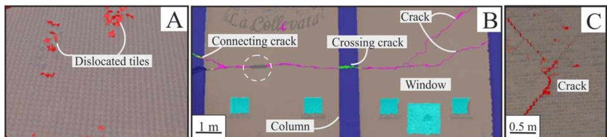
Figure 4: Damage features identified with object-based image analysis (OBIA) in images of a roof with dislocated tiles (A), various damage types on a concrete façade (B), and an image of a brick façade showing extensive cracks.
