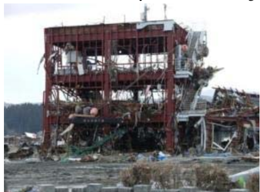
Fig.5 The disaster management center of Minami-Sanriku town (March 23)
