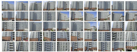
Figure 7 A full view of facades.
