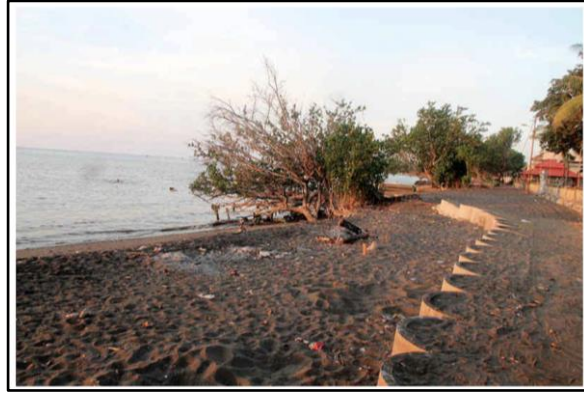
Figure 9. The revetment at Buleleng beach to protecting the coastline from abrasion (Source: Balipost)
