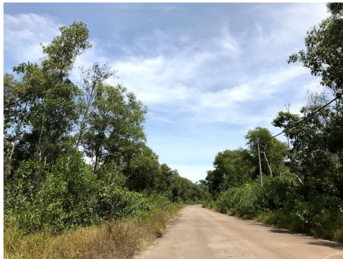
Figure 25: Road Condition in Karambunai
